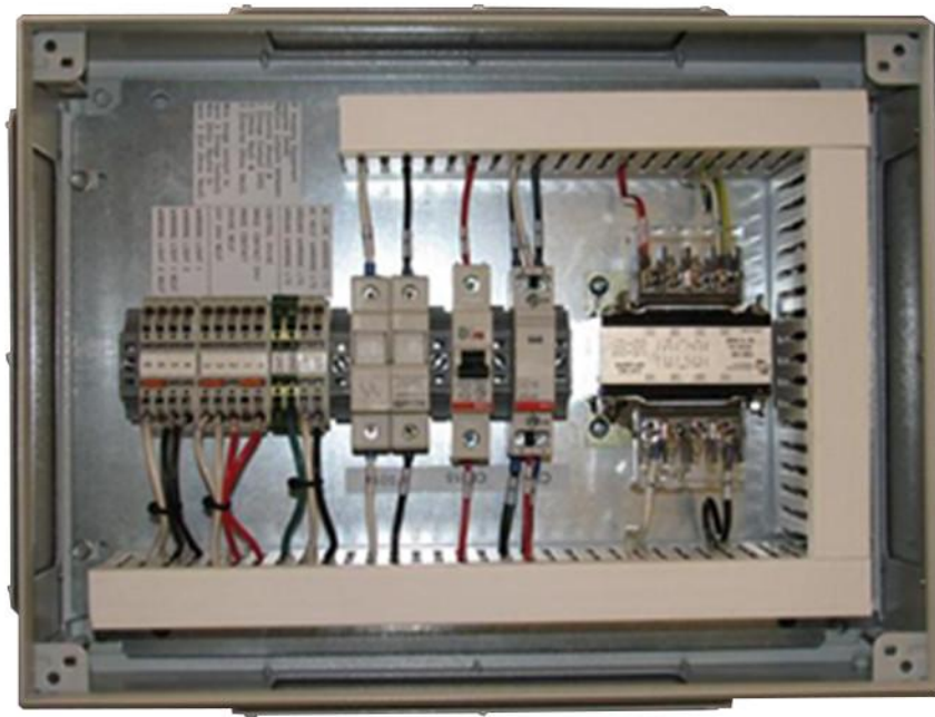
Figure 2 Nova Warning Light Controller- Inside
