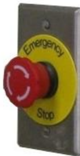
Figure 1 Nova Emergency Power Off Control Station
