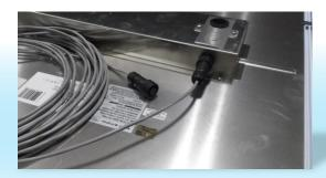
50' cable is connected at LED panel and at Power Distribution Module. No Tools Required.
